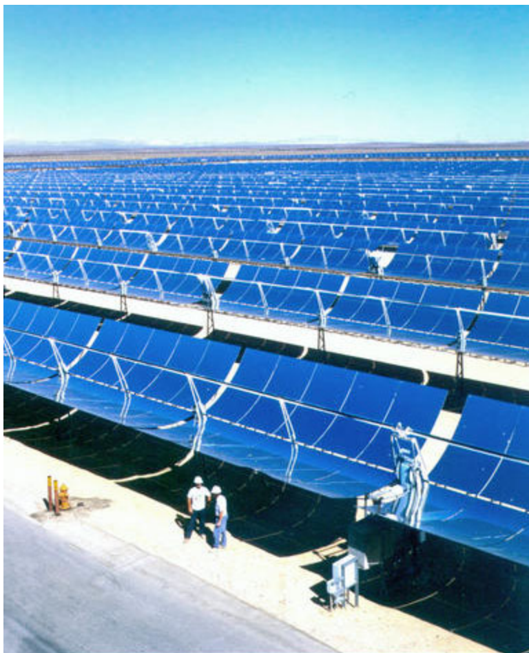
Rows of parabolic mirrors that concentrate sunlight on the tubes in the middle of the mirrors. Oil inside the tubes, which is heated by the concentrated sunlight, is used to generate electrical power.
