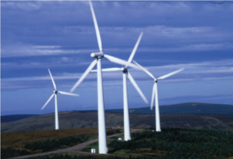
Generating electricity from the wind
