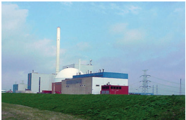
Nuclear power plant in Borssele, the Netherlands.
